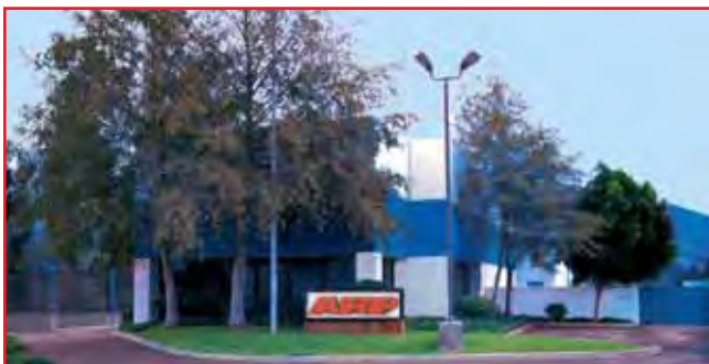
All metal finishing operations are done in this Santa Paula plant.
